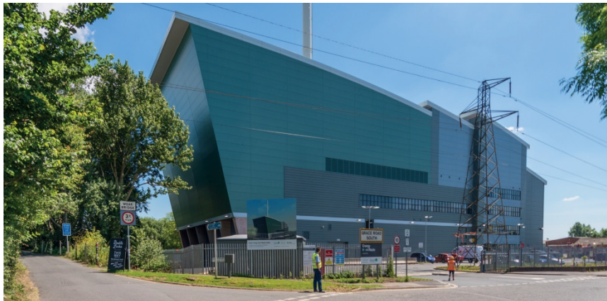
Figure 23: Exeter Energy Recovery Facility
