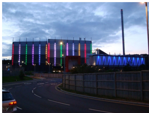
Figure 24: Plymouth Energy Recovery Facility
